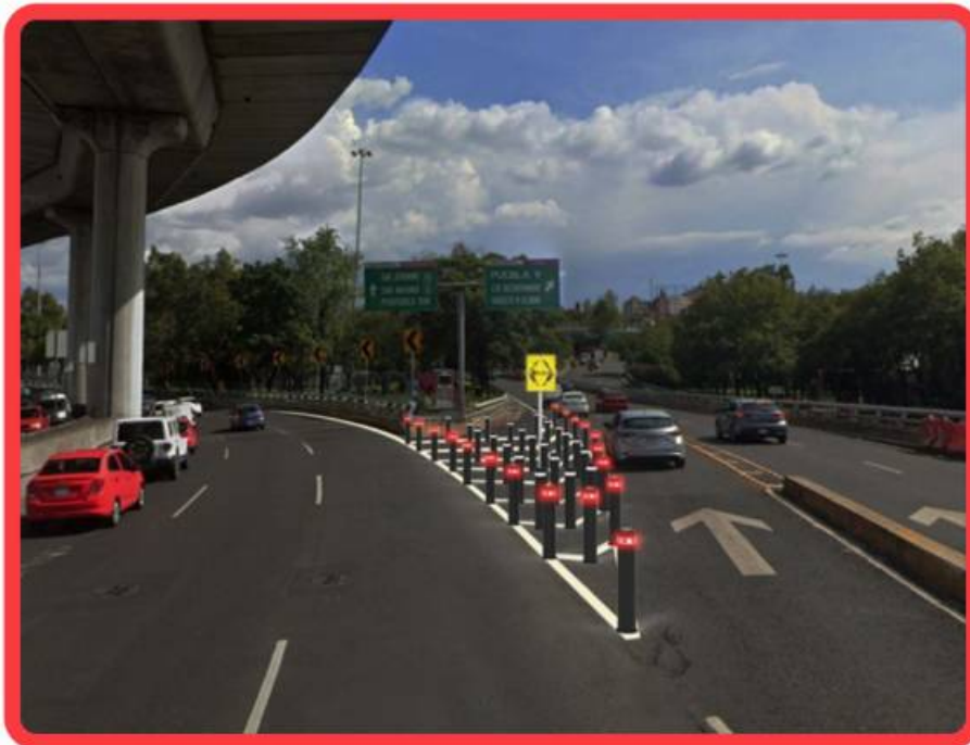
ISLE OF LIFE; Flexible robust inner bollards Arrow sign flexible to impact
