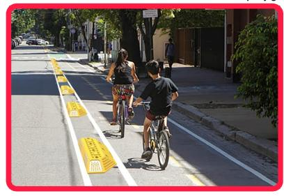
Installation with epoxy 75 glue Steel nail (1/2" × 9.75 in.)
