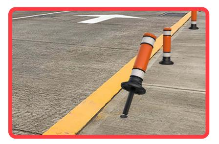
Mark the precise place for make augers on floor. There dig a hole  $\emptyset$  2½" x 12 in. depth.
