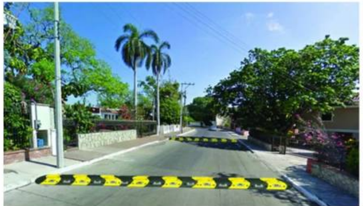
SPEED BUMPH WITH ROAD STUDS
